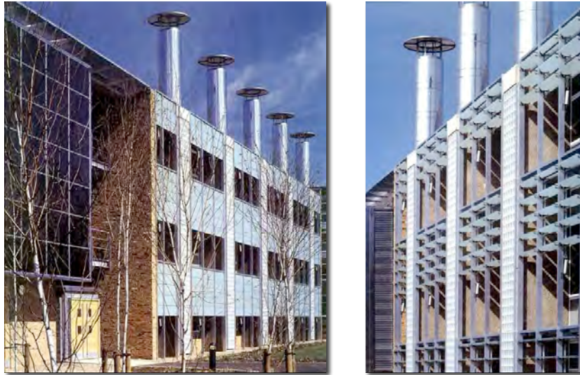
BRE Environmental Building, Feilden Clegg Design, Garston, UK. 1997
