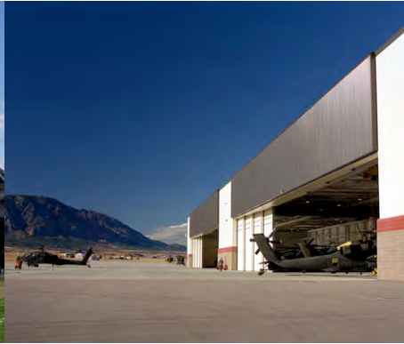
Solar Hot Air
