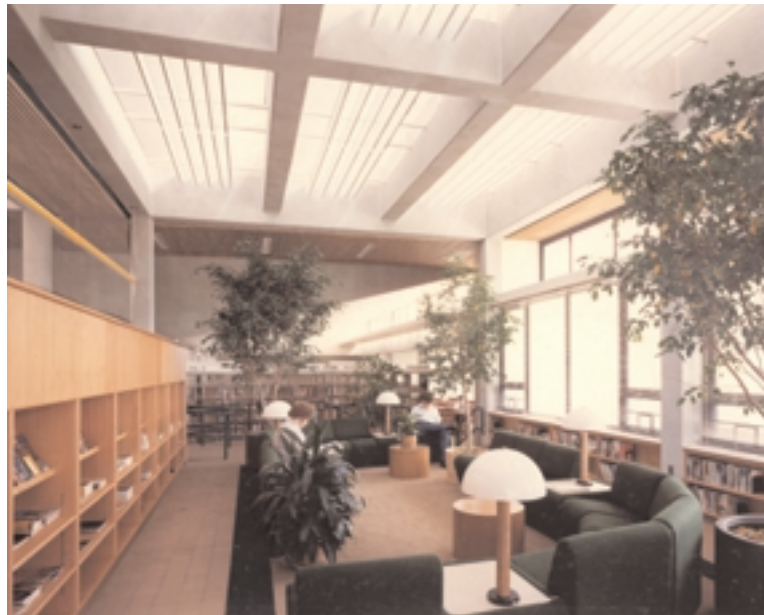
The Mount Airy library, in Mount Airy, North Carolina, a U.S. Department of Energy demonstration project built in 1981, is a completely daylight, passively heated and cooled facility that uses 75 percent less energy than a typical library in the region.
