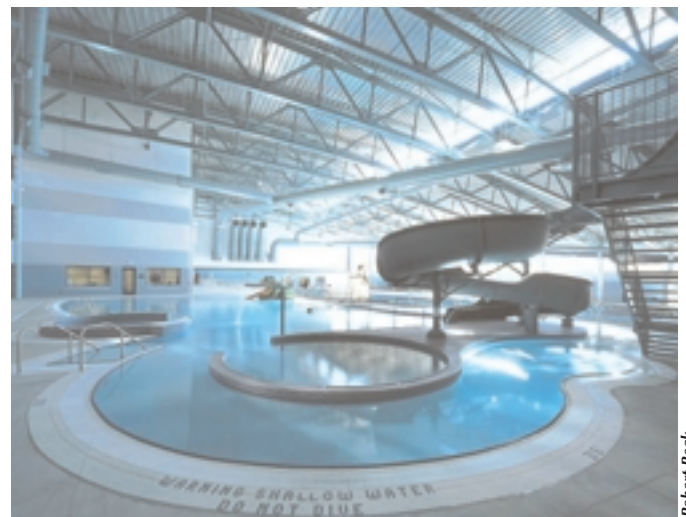
The Natatorium of the 170,000 square foot Genoveva Chavez Community Center in Santa Fe, New Mexico, is a current example of a building that incorporates south-facing clerestories for daylighting and heating, as well as to take advantage of the special quality and intensity of light in Santa Fe.
