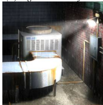
(c) Rooftop light cones
