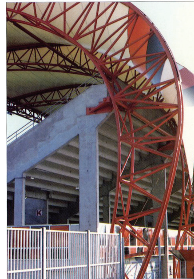
Fig. 213: Racetrack grandstand, France.
