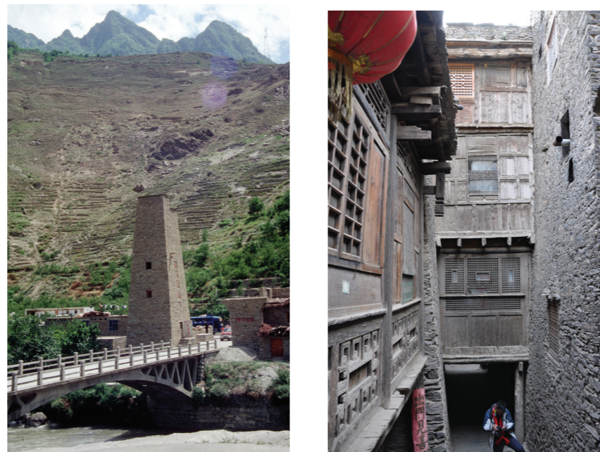
Figure 1.2 (a left) Taoping in its setting with a bridge over the Zagunao River and old-style tower, both recently built (2002); (b right) interior street (2008). Photographs by Dan Abramson.
