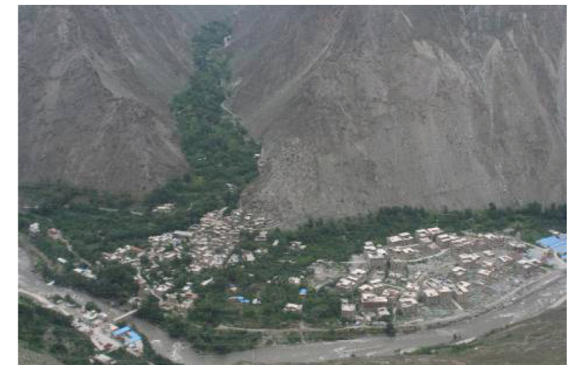
Figure 1.9 Taoping with new tourist village construction aborted after earthquake, July 2009.
