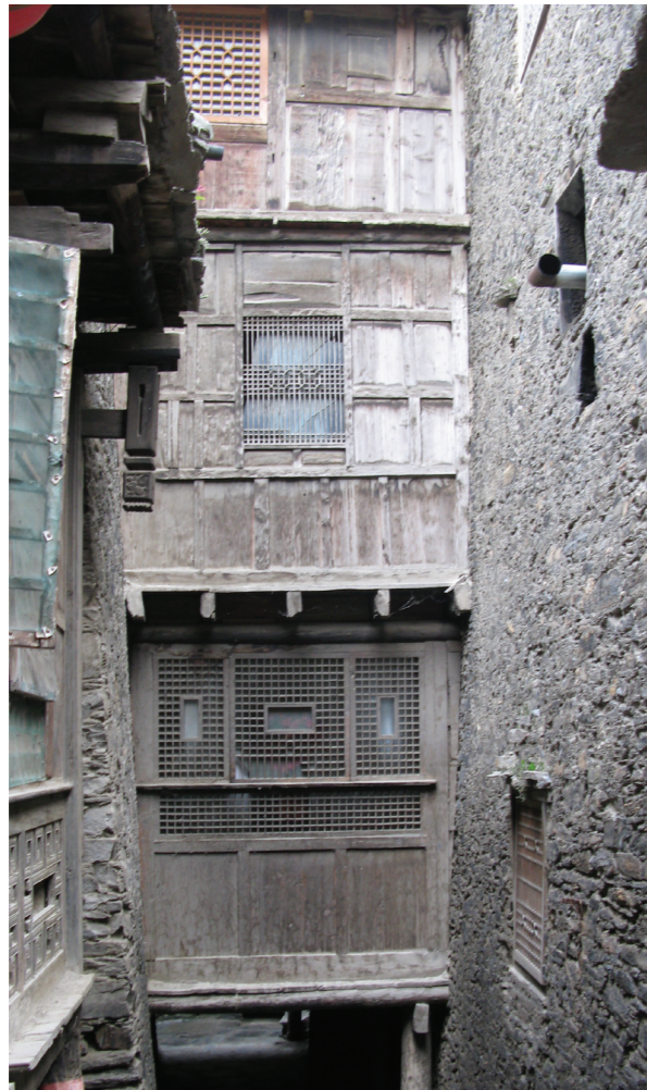
Figure 3.6 Buildings should be reconstructed to their original appearances
