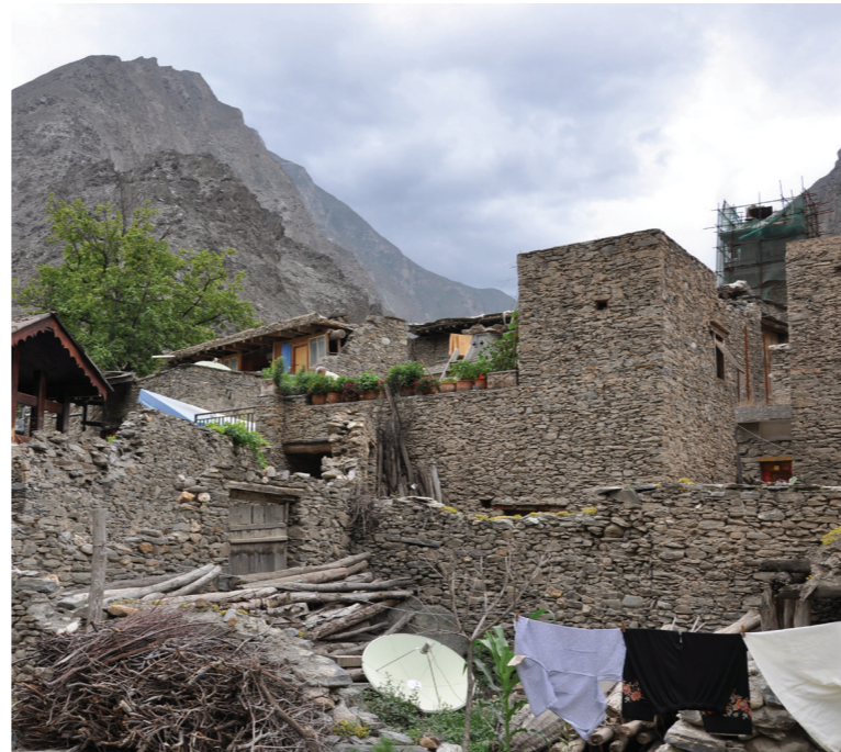
Figure 3.7 New infill development should be allowed if the original structure has sustained severe damage or has collapsed
