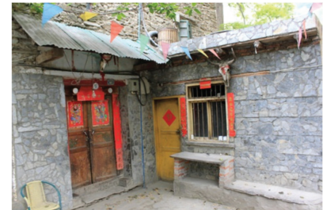
Figure 3.32 Peripheral development with modern materials and larger fenestration
