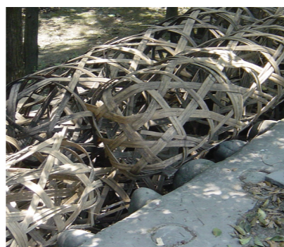
Figure 5.2 bamboo baskets filter slow stream as it joins fast stream at Fish Mouth Levee
