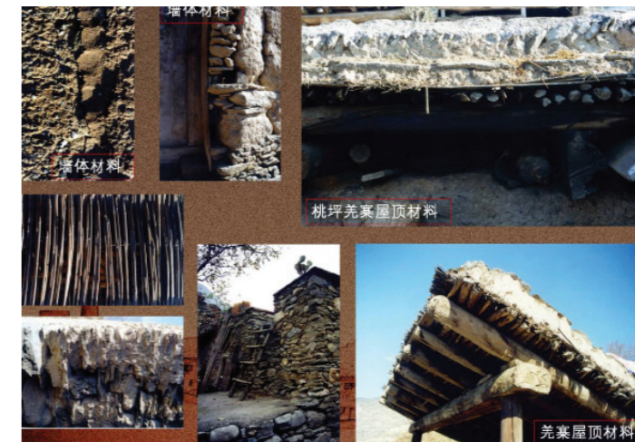
Figure 8B. 4 Integrated roof structure
