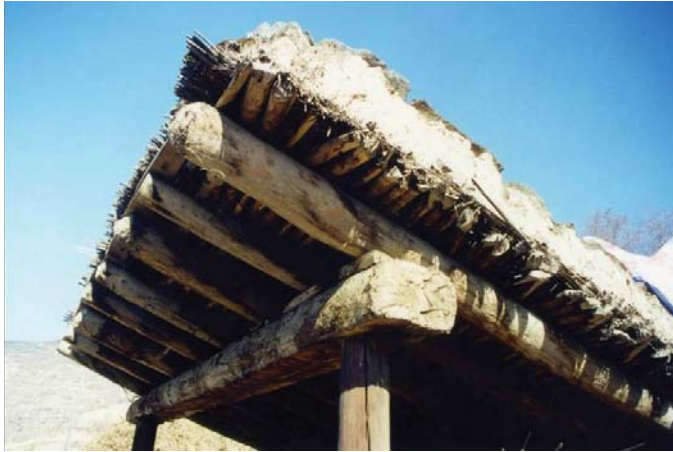
The Qiang people built their houses in multiple layers. For example, this roof has main beams, poles, Citrus medica, and bamboo. On top of the bamboo there is a layer of "Revive Grass" (Selaginella tamariscina), which does not die even after it is dried for several years. When constructing the house, the root of this grass must face up in a layer of mud to absorb water during the rainy season and thereby protect the wooden framework, making it more durable. ( http://www.tudo.com/programs/view/fAaHFLXXOyk )
