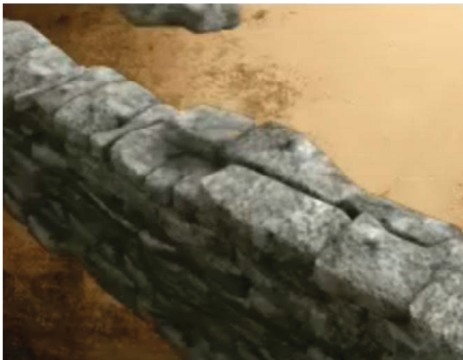
Section of Wall Showing Placement of Bricks, Alternating Directions, CCTV video.
