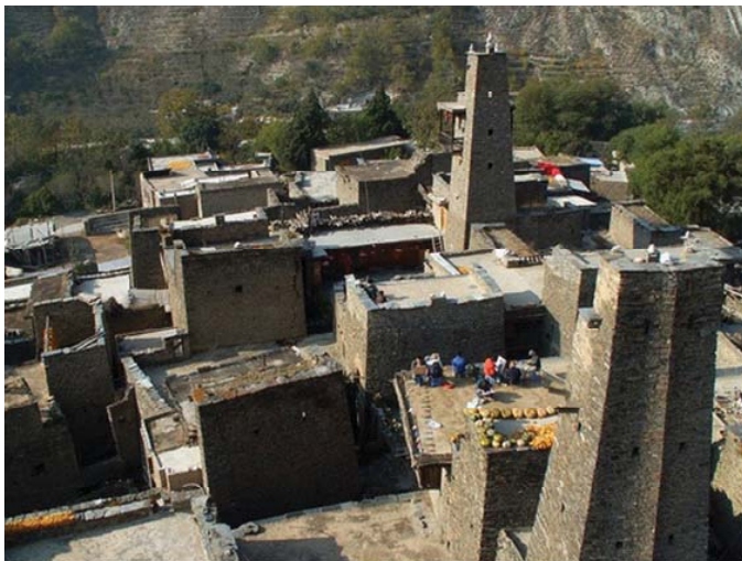
Taoping houses connected in an integrated whole, CCTV video.
