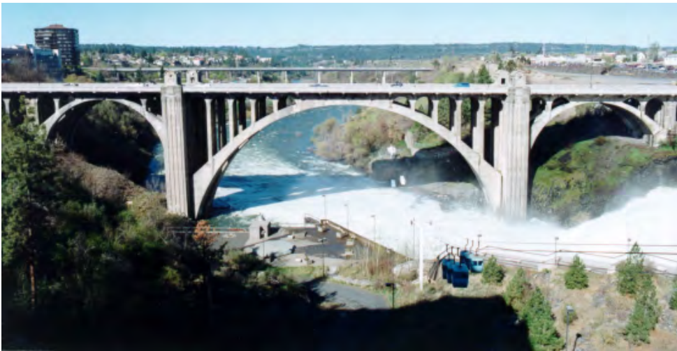
Monroe Street Bridge Restoration Spokane, Washington
