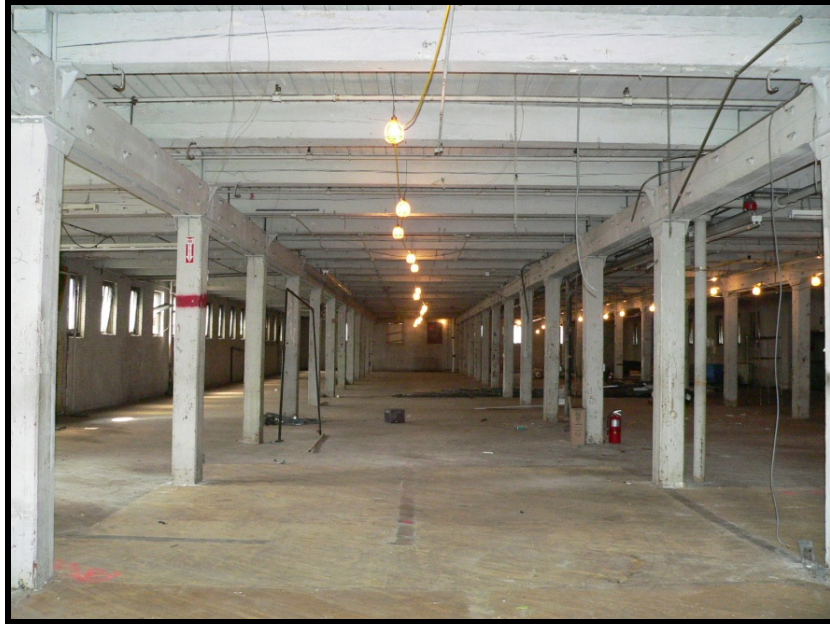
Beam-column-decking system with limited diaphragm action
