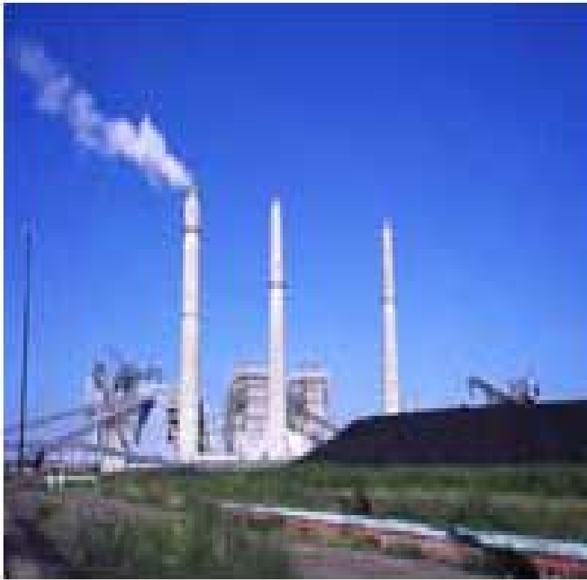
Central Generation Coal Fired Power Plant
