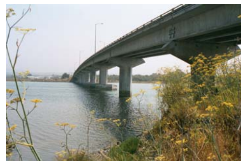
Figure 6. Humboldt Bay Bridge (G. Deierlein photo).
