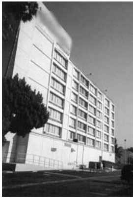
Figure 4. Van Nuys testbed building in 2000 (author photo).
