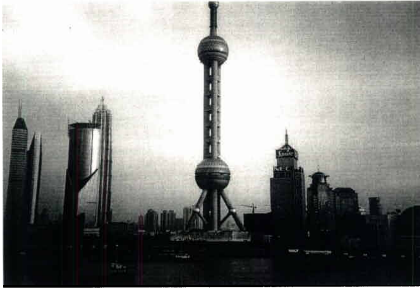
Figure 11.12 In the space of just ten years, Shanghai's new CBD has arisen across the river in Pudong, centered on the futuristic TV observation tower around which modern high-rise buildings have sprung up. Pudong and Shanghai are to be the "Head of the Dragon" in development of the Chang Jiang valley and the rest of China. (Photo by Jack Williams)
