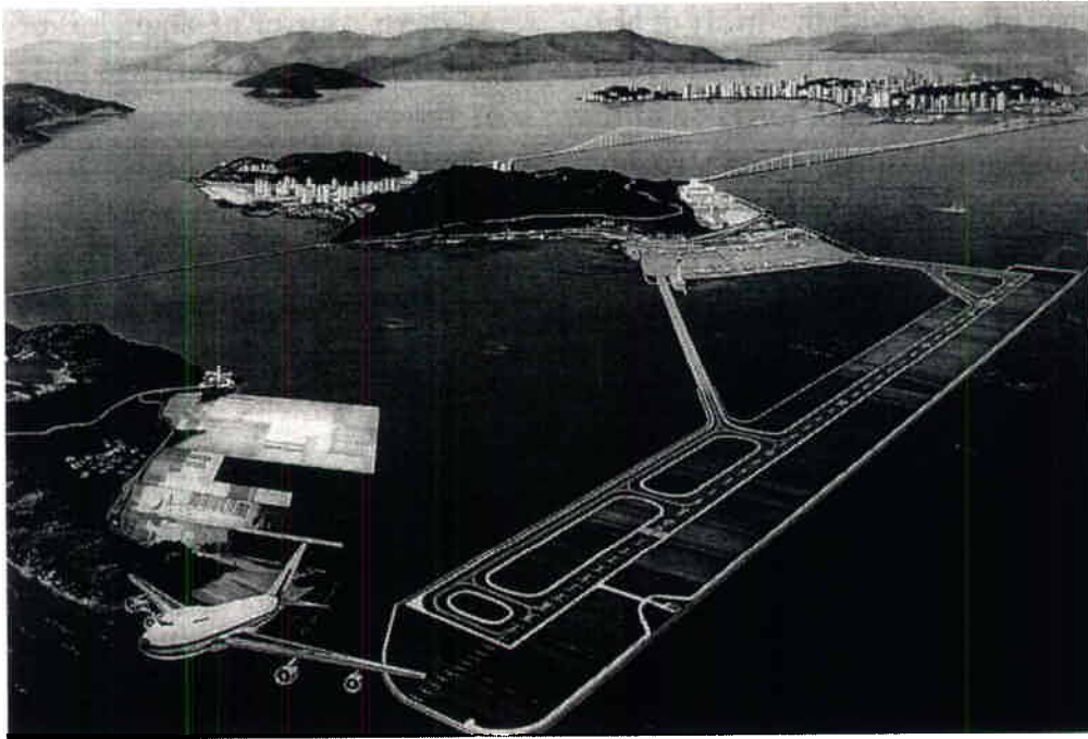
Figure 11.2 Macau's international airport, opened in the late 1990s, stretches on reclaimed land between the two islands of Coloane and Taipa. In the distance, on the peninsula, is the main urban area of Macau. Collectively, these three pieces of land form the Macau Special Administrative Region of China. (Photo courtesy Macau government)
