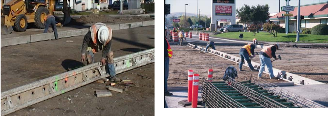
Figure 3 - Steel modular forms being used in concrete pavement construction
