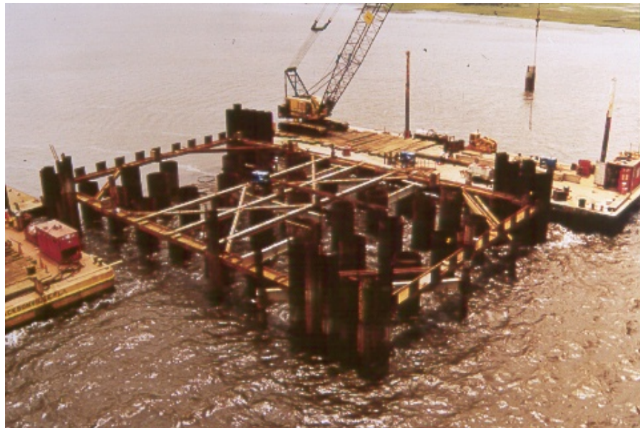
Figure 11 – Installation of wale and strut system
