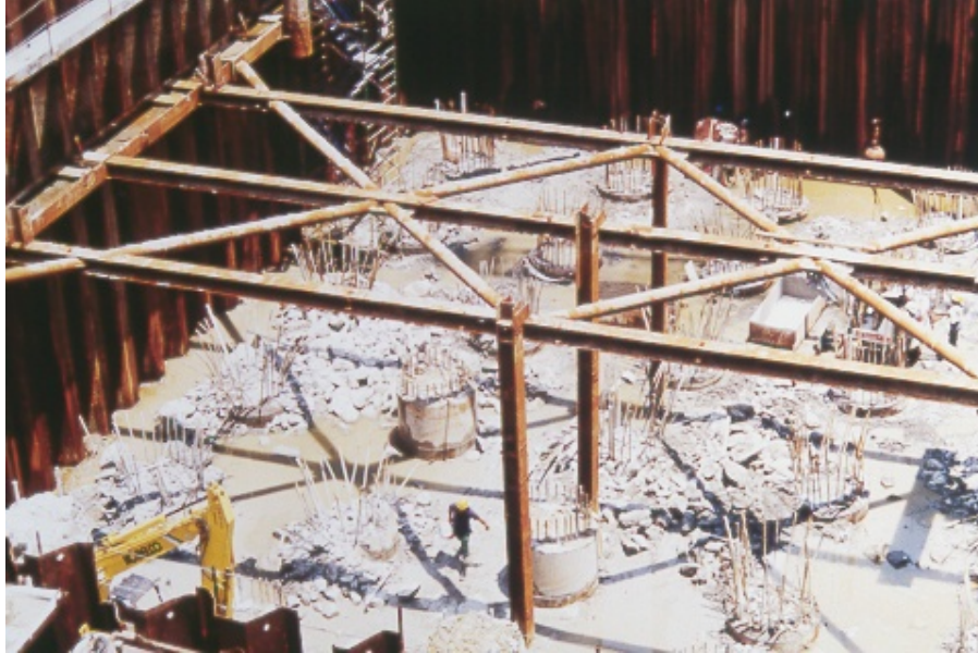
Figure 10 - Cofferdam for the Sidney Lanier Bridge, Oregon
