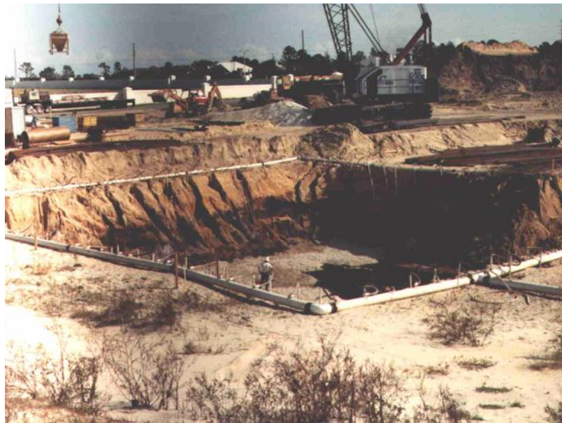
Figure 9 – A typical well point system dewatering
