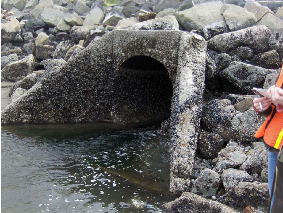
Figure 17. A culvert serves as the exit point of Puget Creek, found in AUW3. (Photo by Canyon Little)
