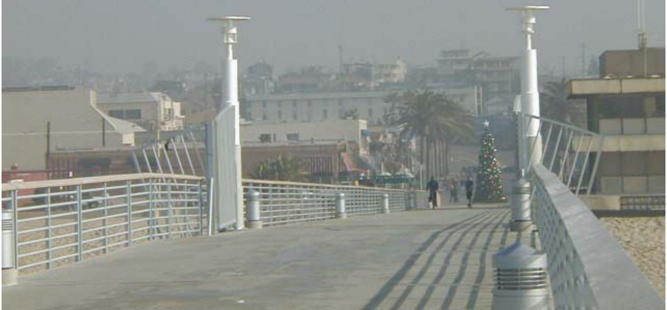
Figure 16: Hermosa Pier Access Gate
