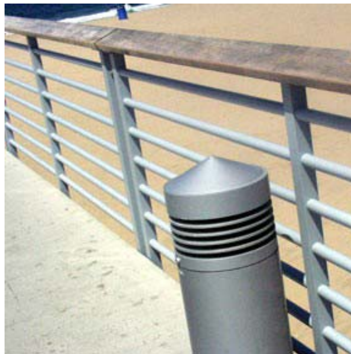
Figure 18: Example Railing System.
