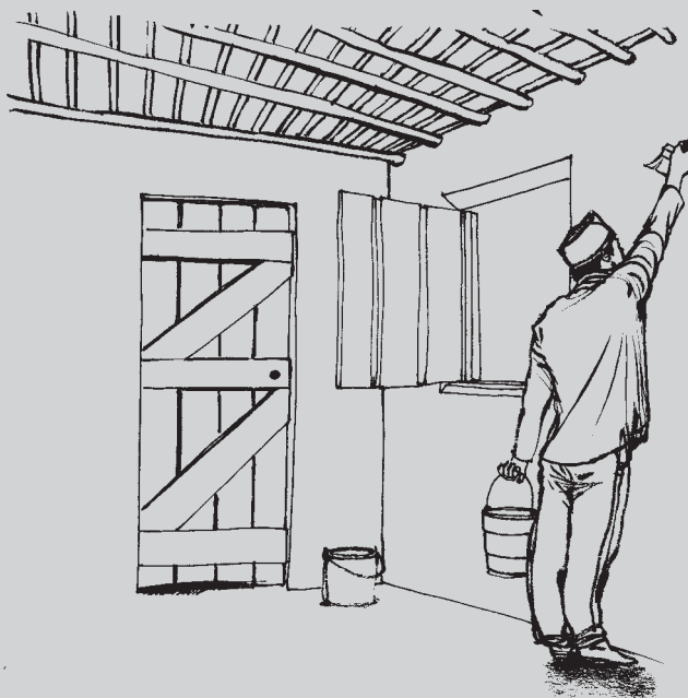
Fig. 1.90 Insecticidal paint can be applied with a brush.
