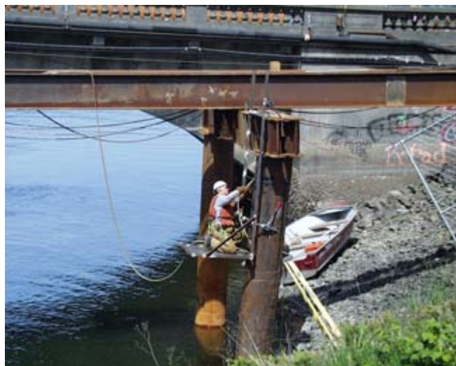
Worker wearing PFD, eye protection, hand protection, and head protection while welding.
