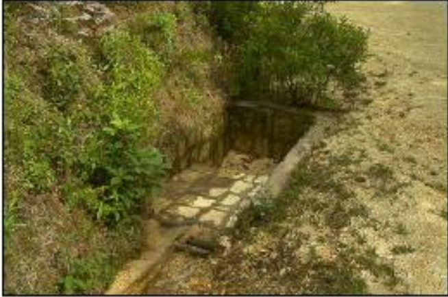
Photo 7.8 Use masonry, concrete, or metal inlet structures to control water in the ditch, direct the water into the cross-drain pipe, and prevent ditch down-cutting.
