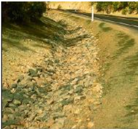
Ditch line armored with angular rock to withstand erosion
