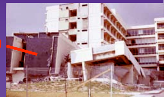
Olive View Hospital San Fernando quake, 3 out of 4 fell over
