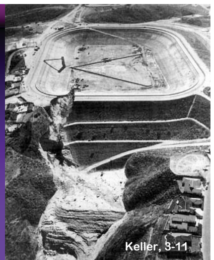
View of dam after failure
