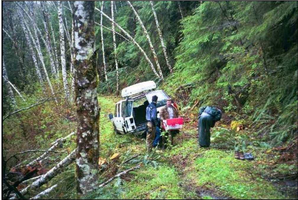
Figure 25 The suburban is stuck in a slump in the roadway caused by problems in the subgrade.
