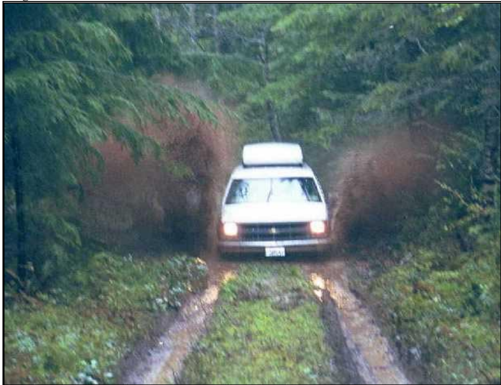
Figure 26 The suburban is driving through a puddle formed on the roadway caused by poor drainage and deep wheel ruts which channel water flow on the road bed. Substantial ballast may be required to provide a suitable traveling surface.
