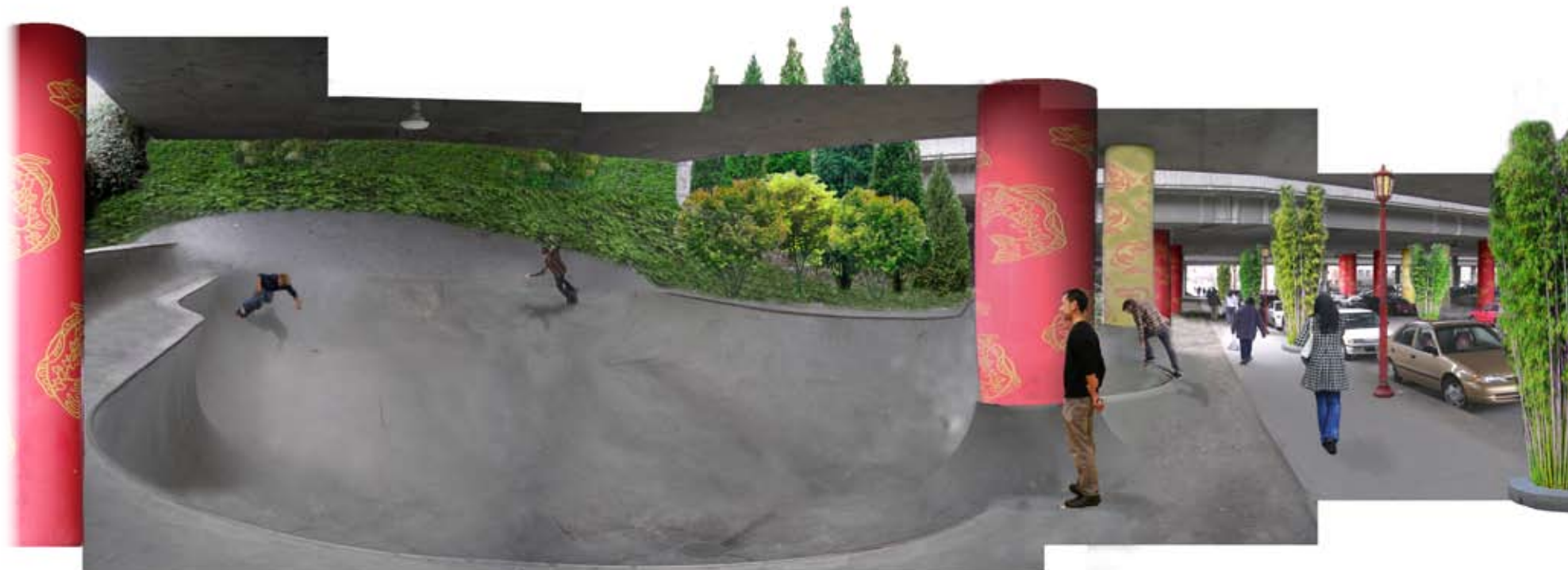
Skatepark takes shape under East side of freeway, on South side of King Street
