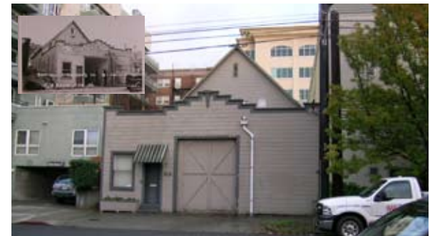
516 Yale Avenue North, a 1905 wood-framed commercial building.
