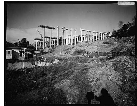
1961 photograph of Lakeview overpass under construction.
