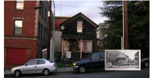
1206 Republican Street, an 1890 worker's cottage.
