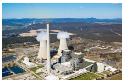
• Vattenfall coal-fired Schwarze Pumpe power station in Germany, a 30 MW oxycombustion CO 2 capture system
