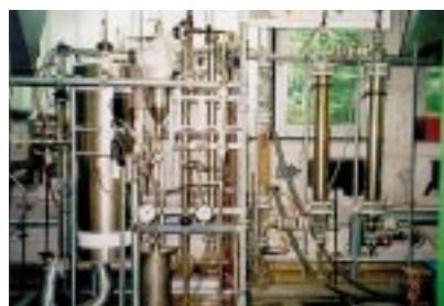
Figure 8: 6 kg/h Fluid bed unit at IWC, Hamburg, Germany
