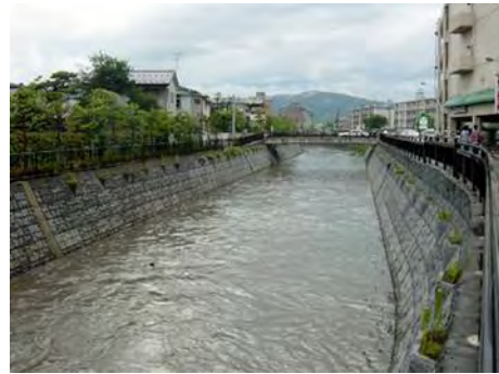
Fig 4 The downstream that have been repaired
