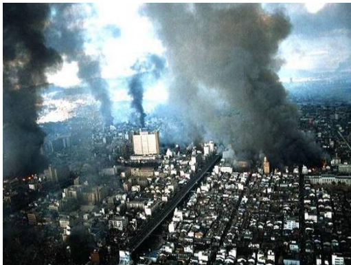
Fig.1 Damage from the Great Hanshin Awaji earthquake (offered by Kobe City)
