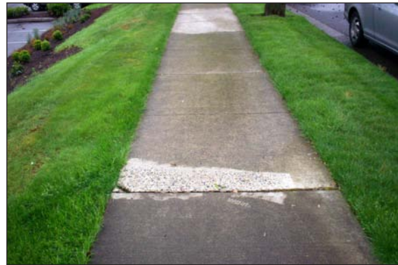
Figures T-20, T-21. Sidewalk repair using the grinding method in Redmond, Washington. Source: UDP Studio.
