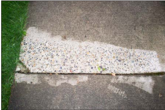
Figures T-20, T-21. Sidewalk repair using the grinding method in Redmond, Washington. Source: UDP Studio.
