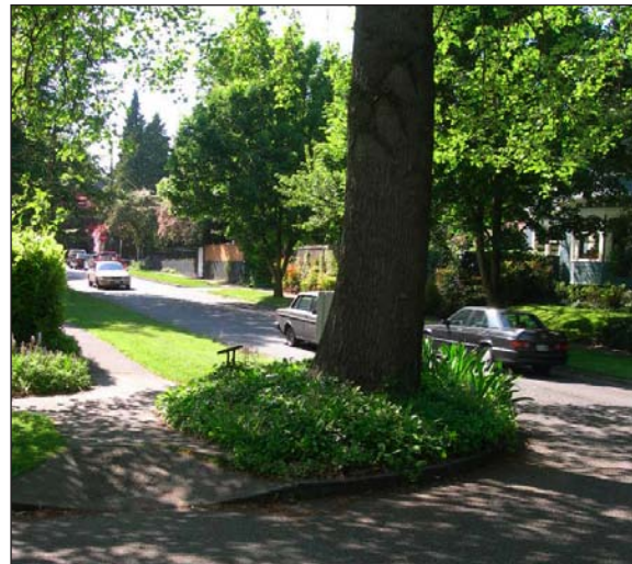
Figure T-19. Sidewalk Repaved Around Tree. Sidewalk designed to accommodate growth of mature street trees. Source: UDP Studio.
