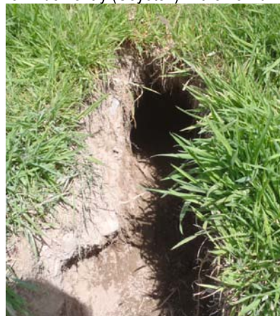
Unknown den entry (Coyote?) in the new dike wall
