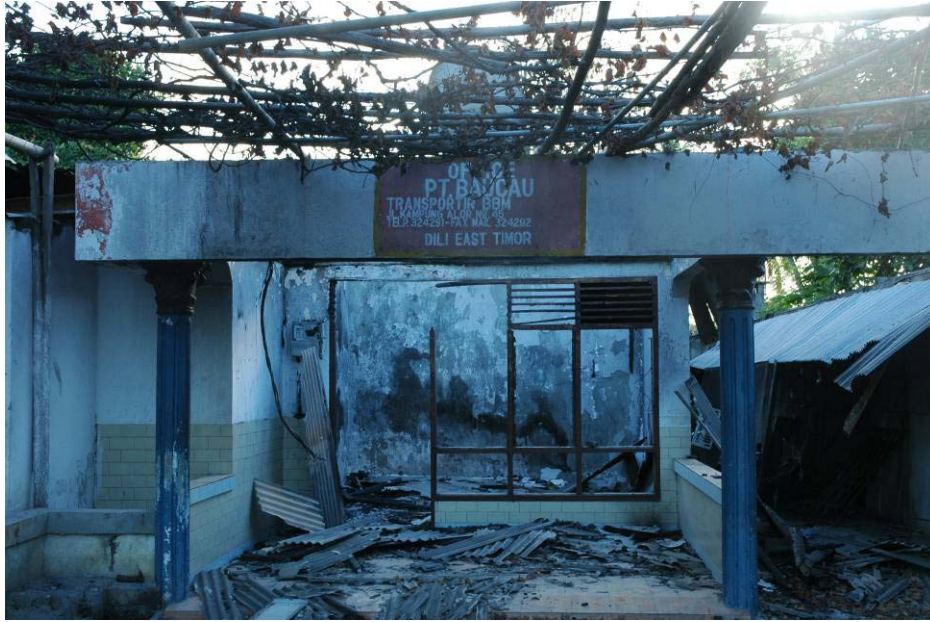
Figure 3 Wreckage of Eastern owned fuel transport business, Kampung Alor
