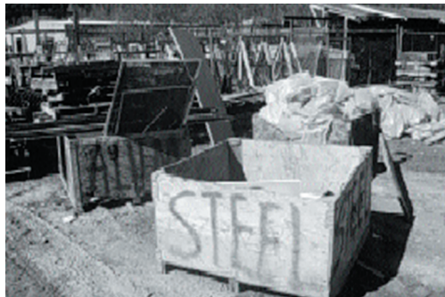
Construction Recycling Photo via http://www.umich.edu
