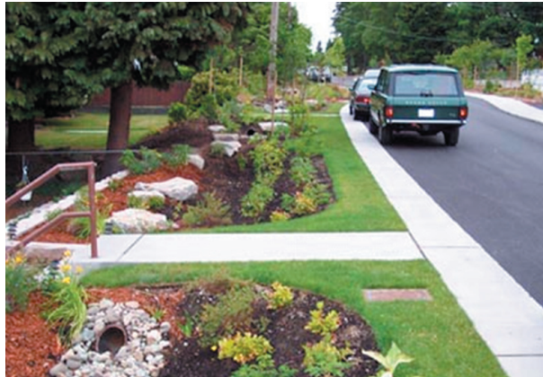
SEA Streets natural drainage system. http://www.seattle.gov/util/About_SPU/Drainage_&_Sewer_System/Natural_Drainage_Systems/Street_Edge_Alternatives/index.asp
