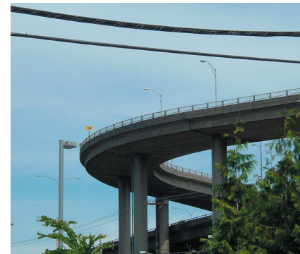
Figure 1.1 The top of the Lakeview Boulevard bridge over Interstate-5
