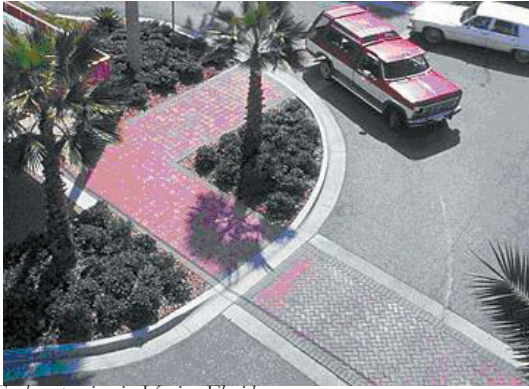
Curb extension in Venice, Florida
