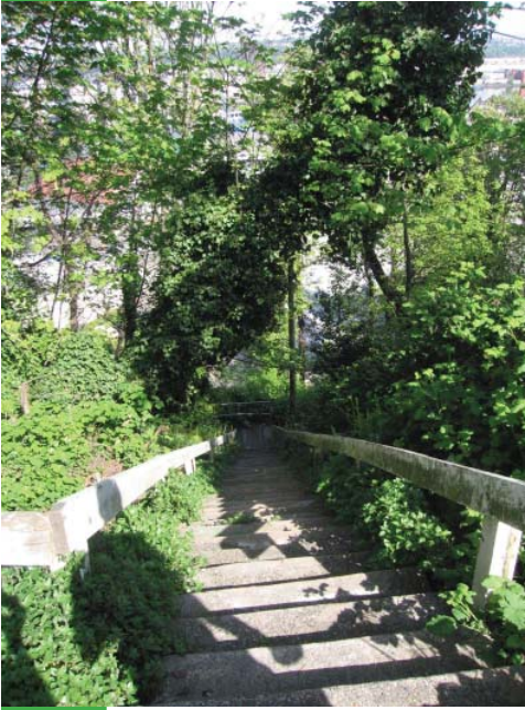
Figure 2.9: Photo from the Charlestown Staircase
