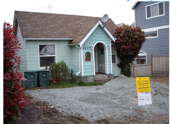
Figure 3.18 New Townhouses in construction 4716 Delridge Way SW
