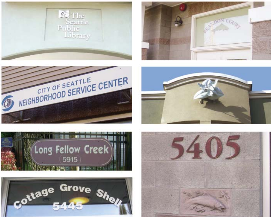
Figure 5.27: Various building features play a part in wayfinding, from addresses and names to artistic elements,
