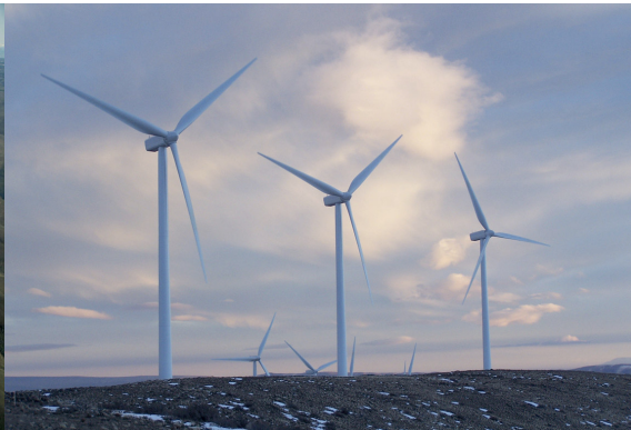
Figure 2 Wind Turbines at Wild Horse [5]
