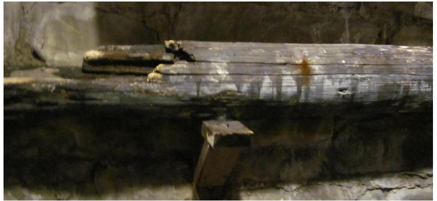
Figure 3: Side View of a Wooden Pipe
