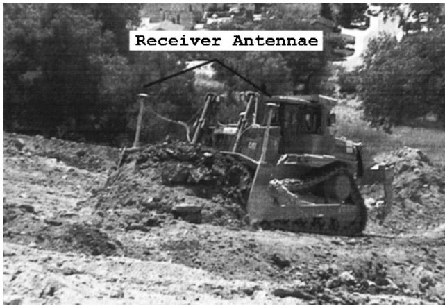
Fig. 4. Caterpillar D9R equipped with SiteVision GPS
