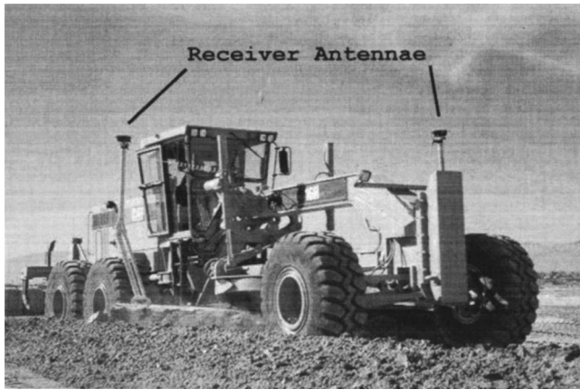
Fig. 2. Caterpillar 16H with SiteVision GPS system (courtesy of Trimble Navigation, Ltd.)
