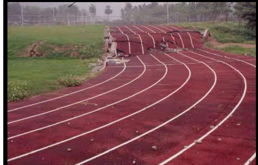
Reverse fault (Chelungpu fault) cutting running track Text, fig. 3-8b RSY
