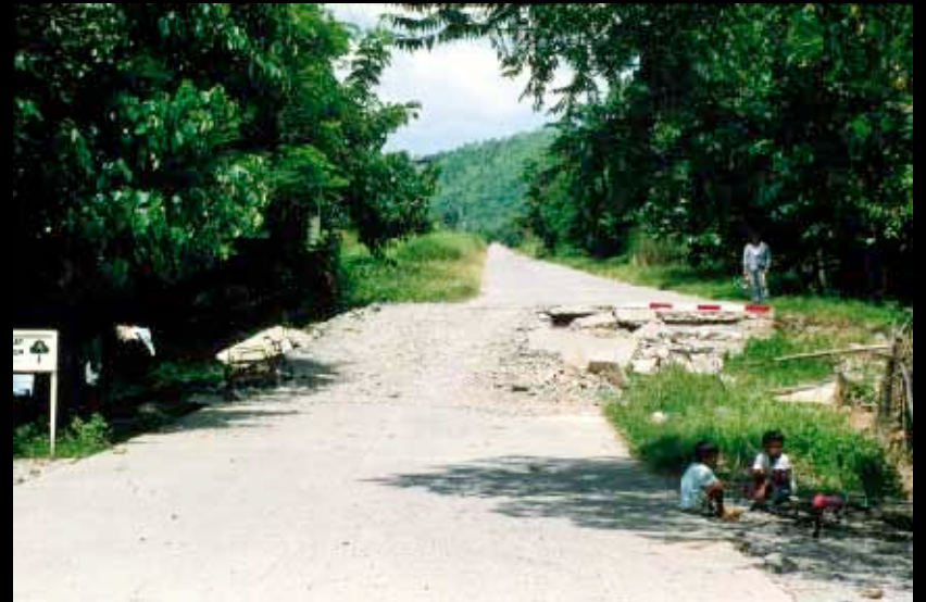
Road offset right laterally by Digdig fault in 1990 (T. Nakata)
