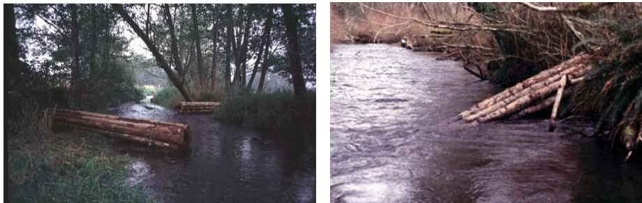
ELWd™ structures installed as ramp logs on Newaukum and Griffin Creeks
