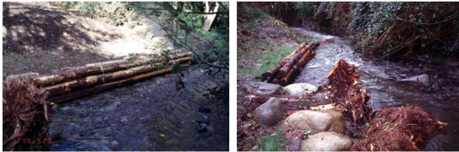
An ELWd™ structure was installed for bank protection at the mouth of a tributary on Thornton Creek.
