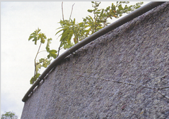
Plastic panels and felt are attached to the frame, with drip irrigation pipes at the top
