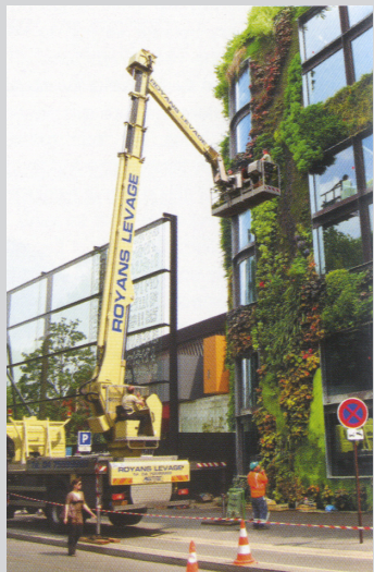
Plants are pruned when they protrude more than 3-4'
