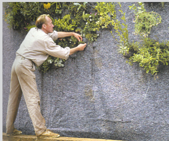
Plants are inserted into slits between the layers of felt
