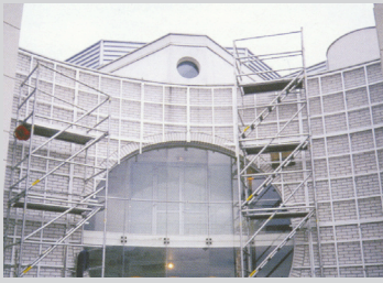
A tubular steel frame is attached to the facade
