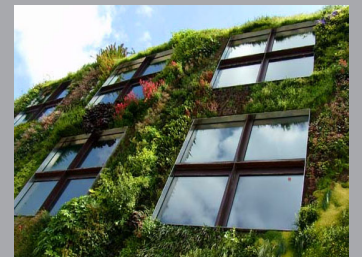
Wall after establishment
