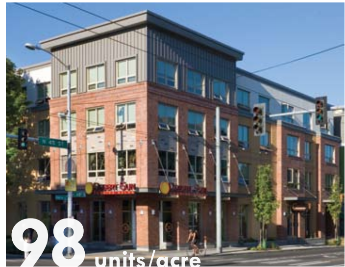
The Stone Way Apartments mixed-use development in Seattle's Wallingford neighborhood provides 70 low-income apartments on 0.71 acres for a net density of 98 units per acre.
