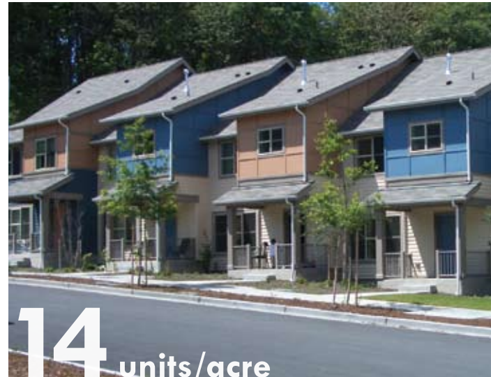
These townhouses at the Rainier Vista mixed-use development in Seattle provide eight low and moderate-income homes on 0.6 acres for a net density of 14 units per acre.
