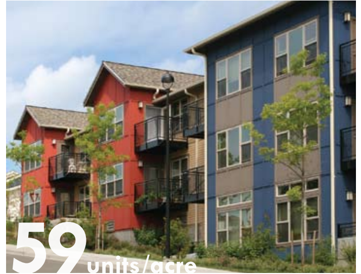
The Nia Apartments at the Greenbridge mixed-use development in White Center provides 82 low-income apartments on 1.39 acres for a net density of 59 units per acre.
