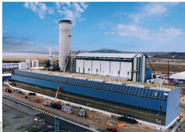
Baglan Bay power station is the launch site for GE's H System ™.
